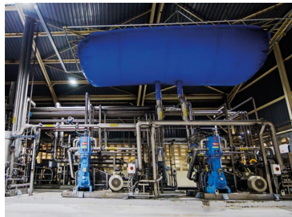
Water treatment technology at one of our facilities in Kenya
