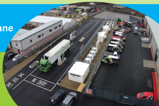
Leyland Bio - CNG Station
