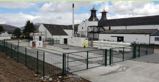
Distillery CNG Daughter Station (above) Offloading Cabinet & Trailer (above, right)
