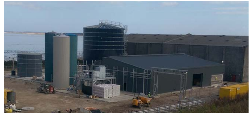
Site progress as at May 2016
